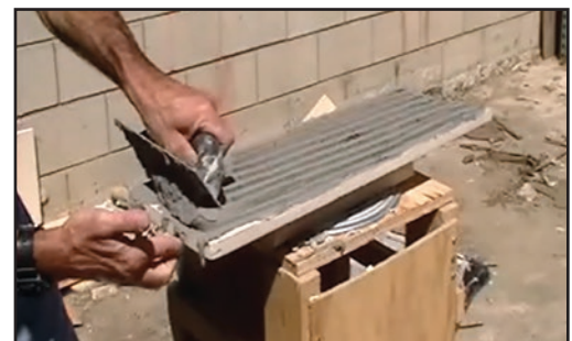
Use a 1/2" notched trowel to apply non-sag polymer-modified mortar to the back of the stone.
